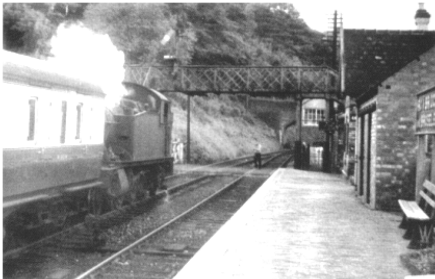
A Shrewsbury bound train leaving Ironbridge and Broseley Station. Note the signalman waiting to hand the token for the section to Buildwas to the Driver
