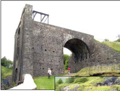
The furnaces were built against a hillside to make charging easier
