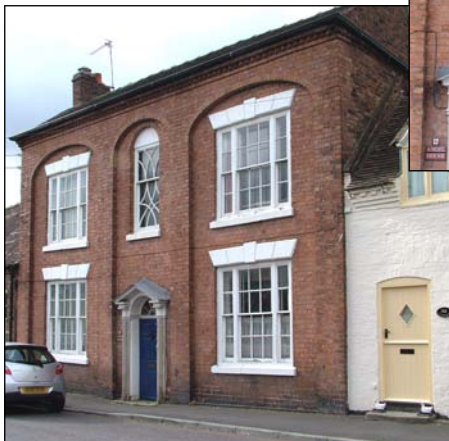
The unusual cast iron window frame above the door of Angel House
