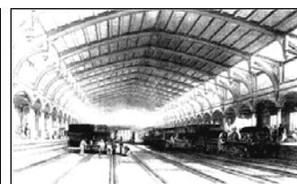
The hammerbeam roof in Brunel's Temple Meads station The newly restored ss Great Britain, floating on her 'sea of glass'
