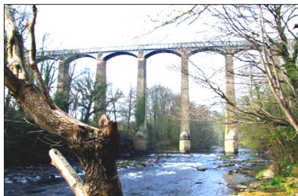
The 'stream in the sky', Telford's 1007 ft span Pontcysyllte aqueduct, which took £47,000 and ten years to build
