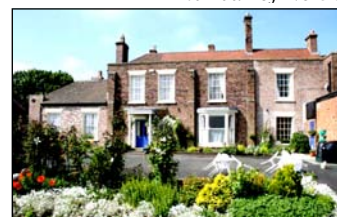
The rear of No 50
