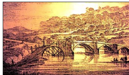
A temporary ferry operated while Buildwas Bridge was being repaired c 1790
