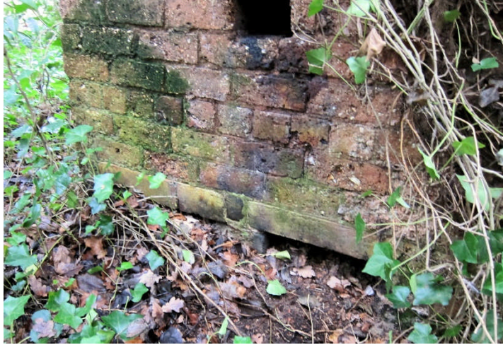
Figure 6. The base of the chimney is constructed of poor-quality bricks. The flues from the drying floor are visible at the base of the chimney.
