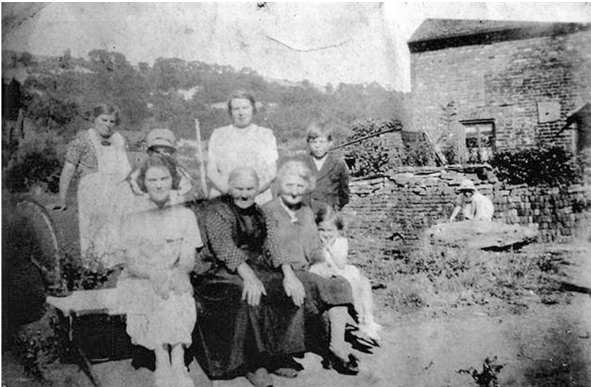
This family group photograph was taken outside the cottage at the Calcutts about 1932. The writer's grandmother is sitting centre front, with her mother, aunt and herself (with hat!) standing behind. Note the cottage wall and also the large old pipe (to the left of the group), a relic of the foundry that once stood here.
