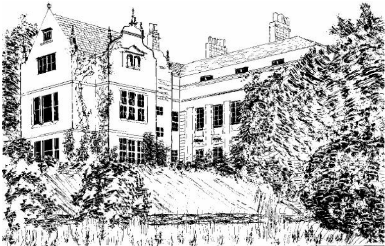
Brymbo Hall. The building was demolished in 1973 when open cast mining was carried out in the area. (Ron Davies)
