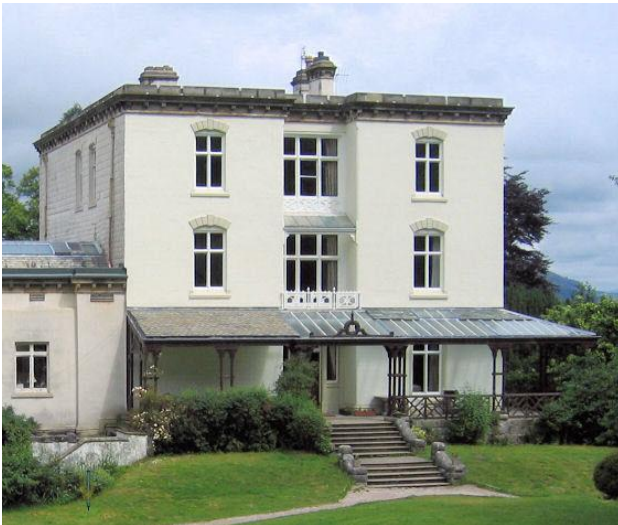
Castle Head with later Victorian verandah. The house is now a Field Centre
