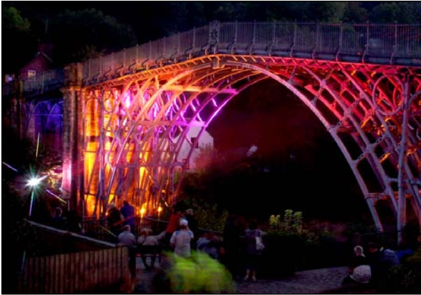
The Iron Bridge all lit up at the Ironbridge Heritage Festival in 2008
