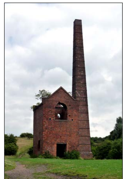
Cobb’s Engine House was built in 1831 to accommodate a Watt beam engine which pumped water from the many deep coal mines that once riddled Bumble Hole and Warren Hill
