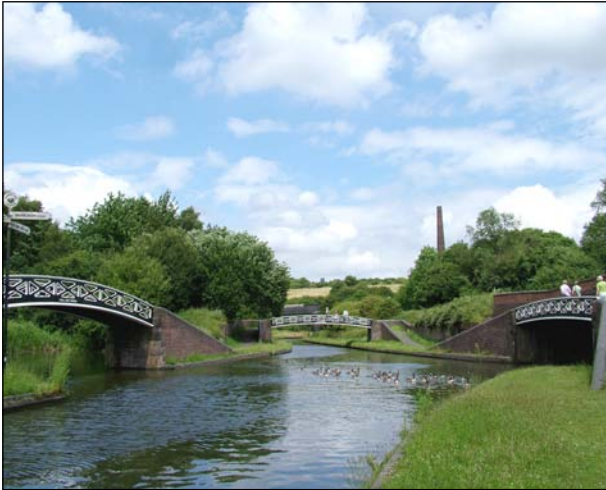
These cast iron footbridges over the canals at Bumble Hole were built in about 1830 at Tipton
