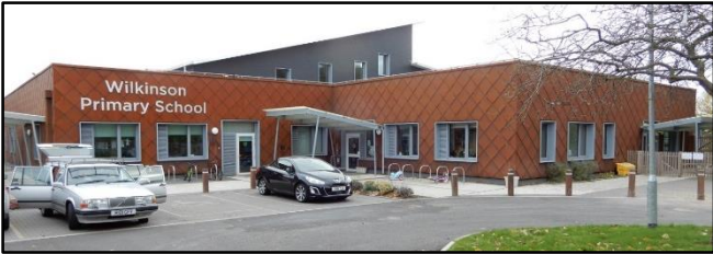
The new Wilkinson Primary School
