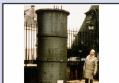
1782 Beam Engine cylinder By courtesy of the Bershram Heritage Museum, Wrexham
